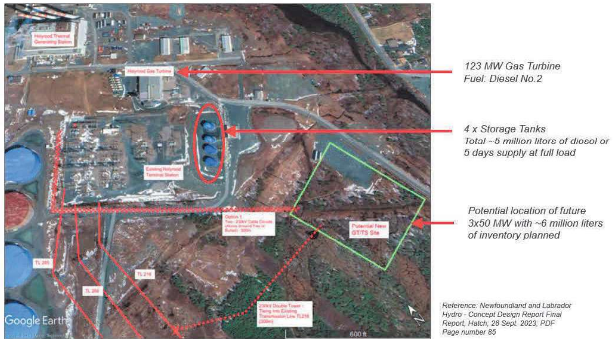
Figure 3 Holyrood Gas Turbine and Storage Tanks: current and proposed (3x50MW)
